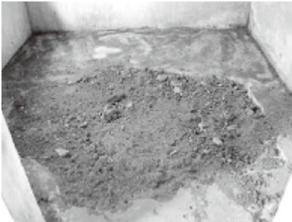
Excavated floor left bare by police forces.
