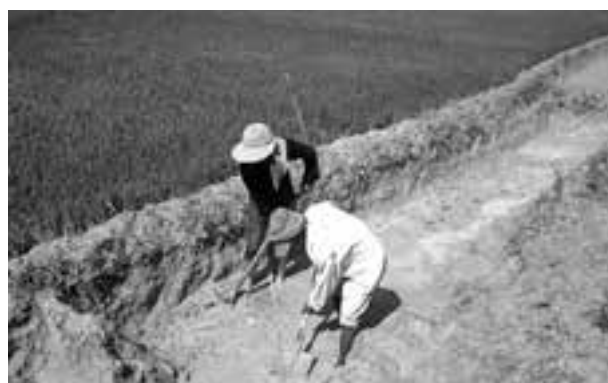
Villagers constructing the canal.
