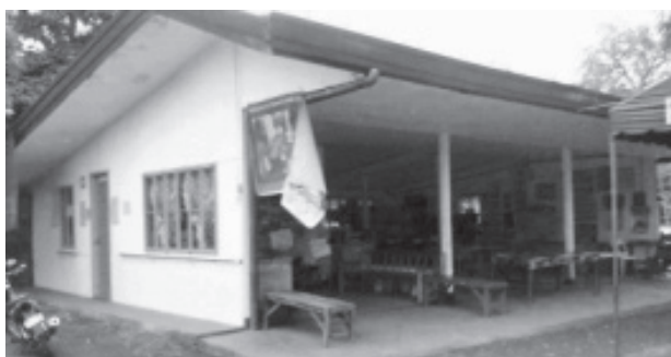
Puan BHS constructed by the LGU.
