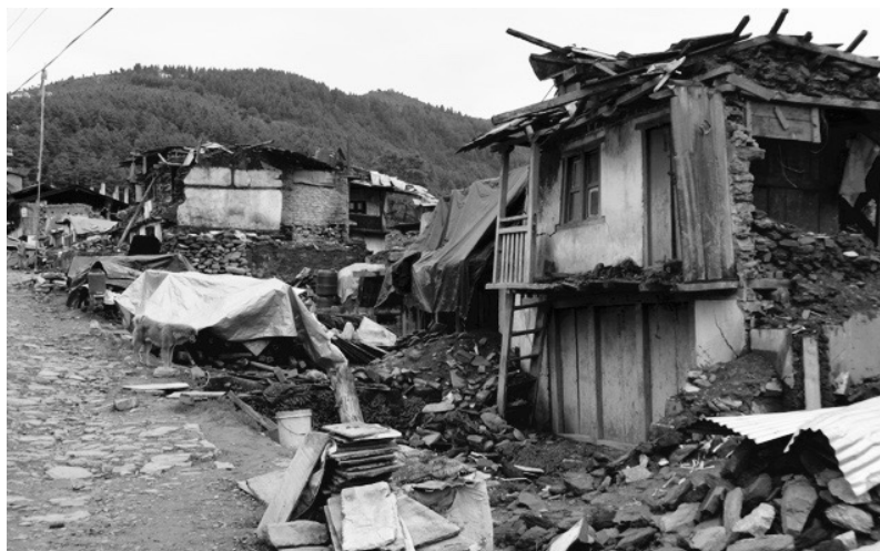
Damaged buildings in Jiri bazaar, Nepal. Photo by NPCS
